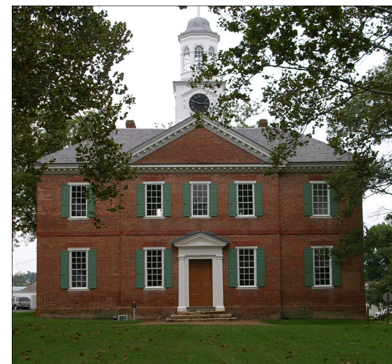
Chowan County Courthouse, 1767 A National Historic Landmark
